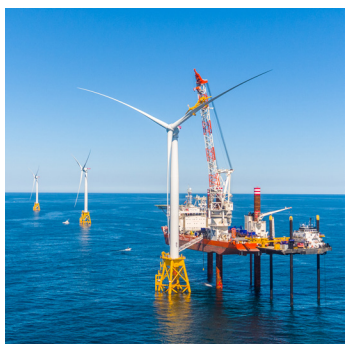
Blade installation, Block Island
