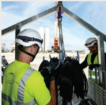
Pre-assembly cabling works
