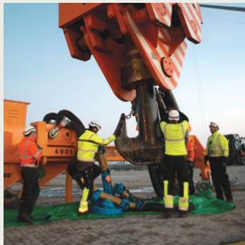
Preparing main hook for lifting operations
