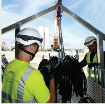
Pre-assembly cabling works
