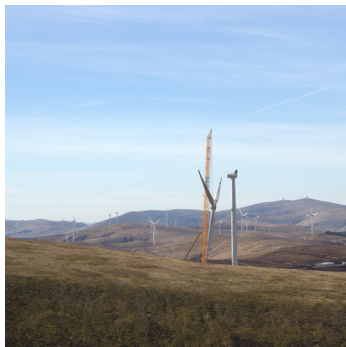
Installation of the rotor-star
