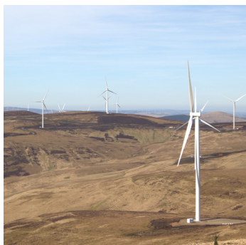
Wind farm overview
